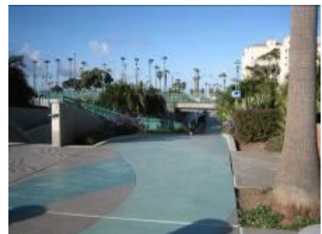
Grade-separated Pedestrian Crossing
