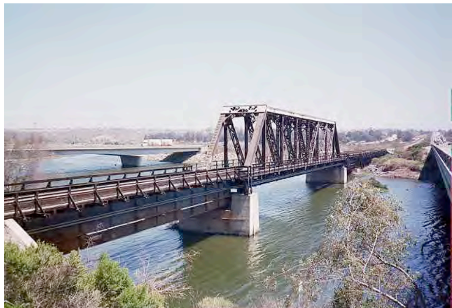
Santa Margarita River Bridge – steel thru-truss and deck girder portion
